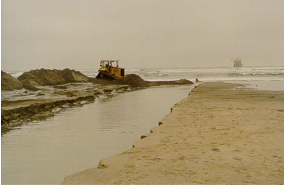
Back-filling cable trench – NorthStar Cable
